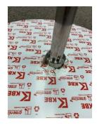
3. Take base section of pole, which has a heavy flange and 3 holes underneath and 3 large Black counter sunk screws. Insert crews through bottom of base plate whilst holding the base section of the pole in position so the 3 bolts can be tightened, securing the pole to the base
